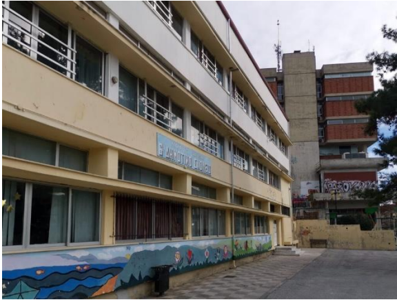
District of Kozani (EL), where renovation works will be carried out.
